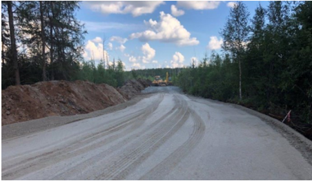
Cleared ROW (Right of Way) area.
