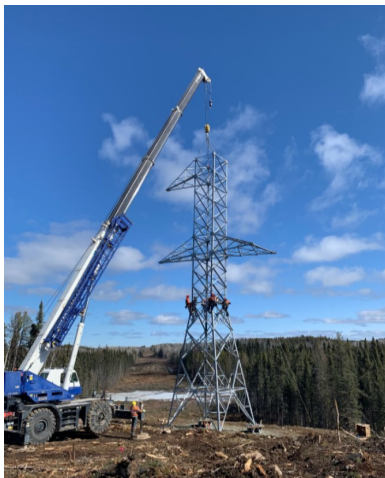
Tower erection progress.
