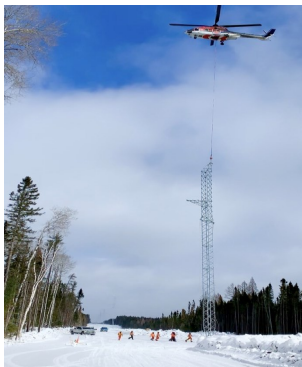
Setting the final Tower
