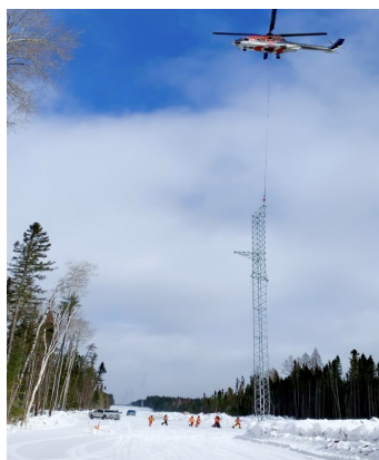
Setting the final Tower
