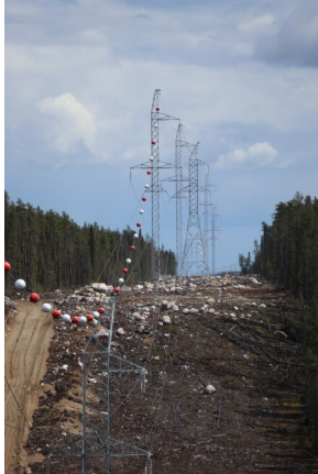
Erected towers along Right of Way between Dinorwic and Pickle Lake
