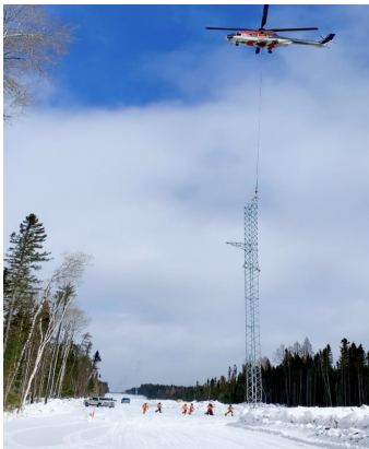
Setting the final Tower
