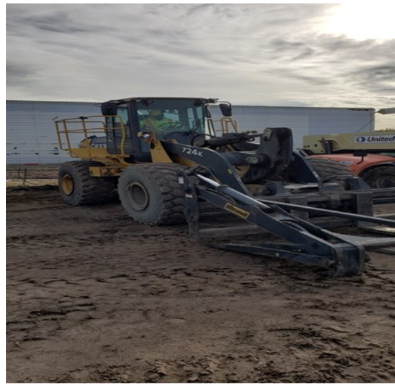
A piece of heavy machinery used on the project
